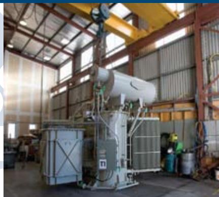
Once fully assembled, the refurbished unit was tested and transported to Harewood for installation and commissioning.
